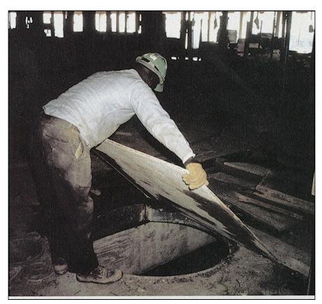
Small openings covered with a single sheet of plywood can be more dangerous than large openings which must be covered with 4x4s and plywood. The reason: a natural tendency when picking up a sheet of plywood is to step forward and into the hole.
