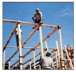
An accident waiting to happen. Walking a 4-inch beam located 10, 12, or 20 feet in the air may seem easy to some workers, but it's definitely not safe. The preferred procedure is shown in the picture on the right.
