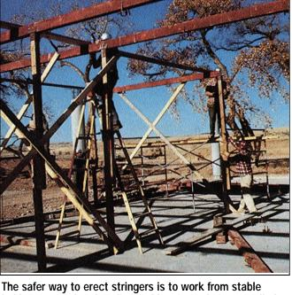
ladders. Note also that diagonal bracing is being installed as the work proceeds, contributing further to stability of the deck forming.
