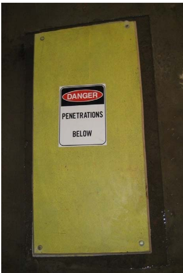
Photograph 4 – Penetration cover showing sign and fixings at each corner.
